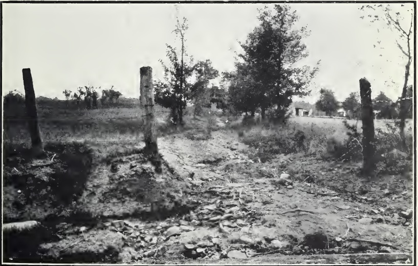
FIG. 2.—DRAINAGE EROSION ON A DRIVEWAY.
